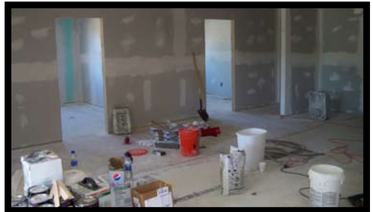
The Princess Palace going through Renovations.
